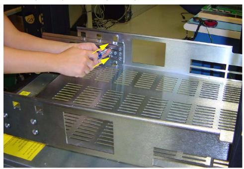
Figure 2-7: Screw the Bracket Into the Shelf From Inside the Rack
